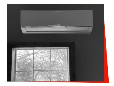
A wall mount is the most common configuration. There is a white rectangular box on the wall however there are a few options beyond the white box in colors. The mounting location is high on an exterior wall so the freon lines can be run through the wall along with the condensate drain.
